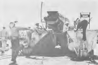
THREE READ-Mix trucks kept concrete hoppers, above, continually filled in the dawn to dusk operation. After a two-cubic-yard hopper, left, was filled, it was swung out to the dolphin by Raymond's big crane, lower left, and dumped in the steel reinforced base, lower right.
